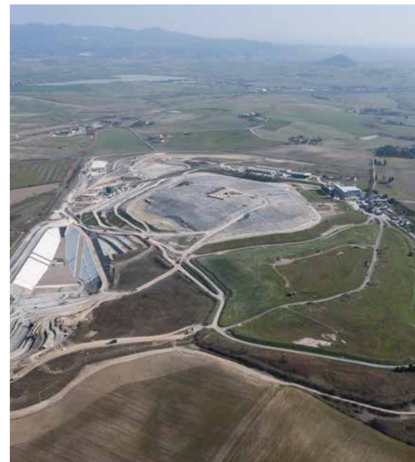
Exe Engineering. Sede a Poggibonsi (Siena)
